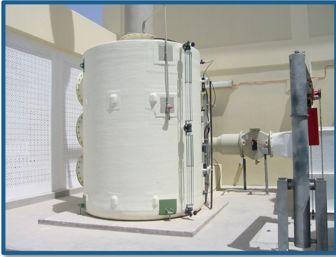
Activated Carbon Unit
